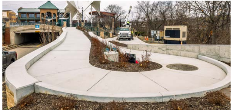
Current progress including new pedestrian connections are now open.
