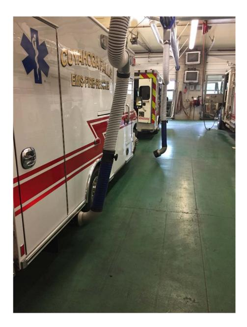
We have recently installed an exhaust capture system (pictured above) to "capture" the exhaust fumes from the vehicles while they are running. The arm automatically ejects from the vehicle as it drives away. The fire fighter reconnects the arm once they arrive back at the station house.
