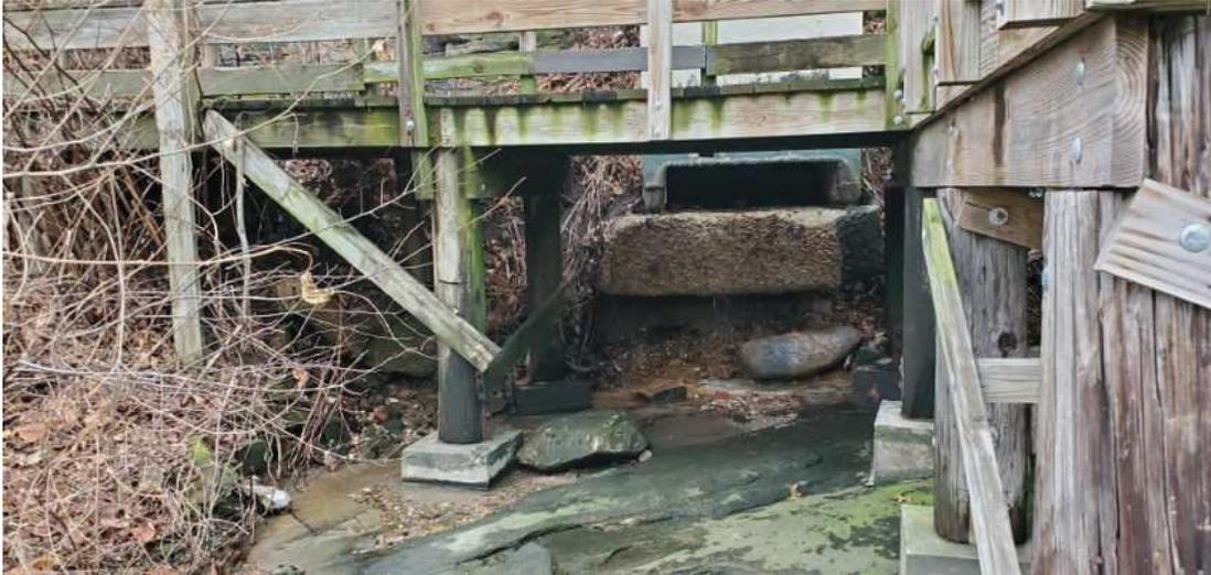
Figure 4: Shallow post footings do not appear to be embedded into the rock.
