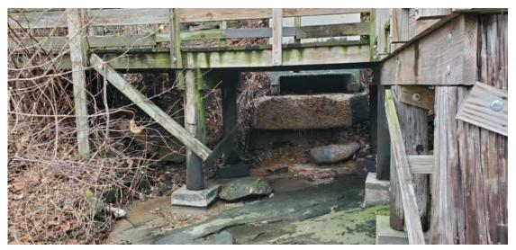
Figure 4: Shallow post footings do not appear to be embedded into the rock.
