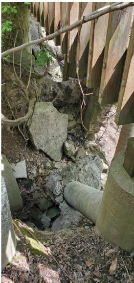
Figure 3: Make shift stone wall above storm discharge
