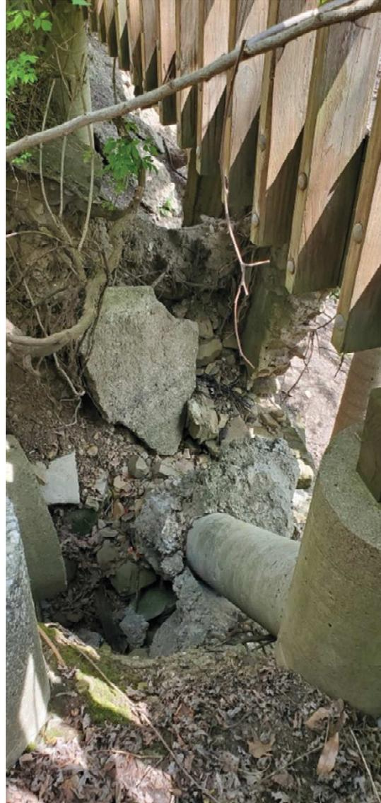
Figure 2: Erosion from storm discharge at upper slopes
