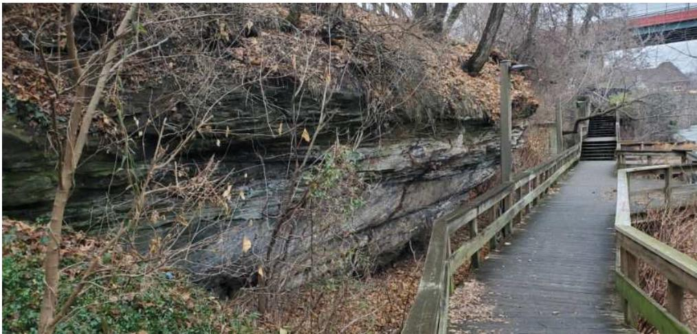
Figure 5: Sandstone with weak non-durable Shale interbeds.
