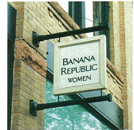
externally illuminated dimensional letters applied to sign panel
