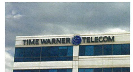
internally illuminated pan channel letters w/ acrylic faces
