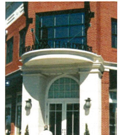
externally illuminated canopy-mounted, dimensional letters
