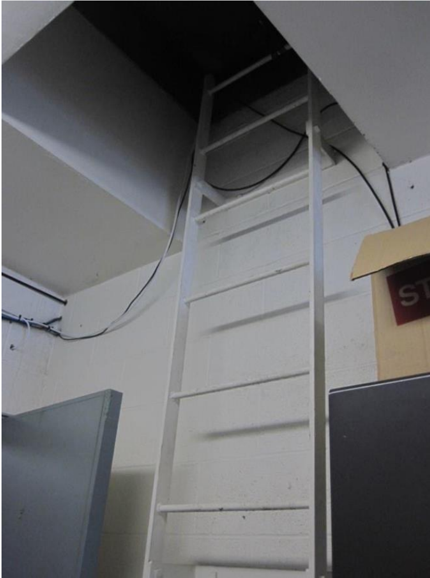
ARCHITECTURAL PICTURE 4: Ladder access to roof
