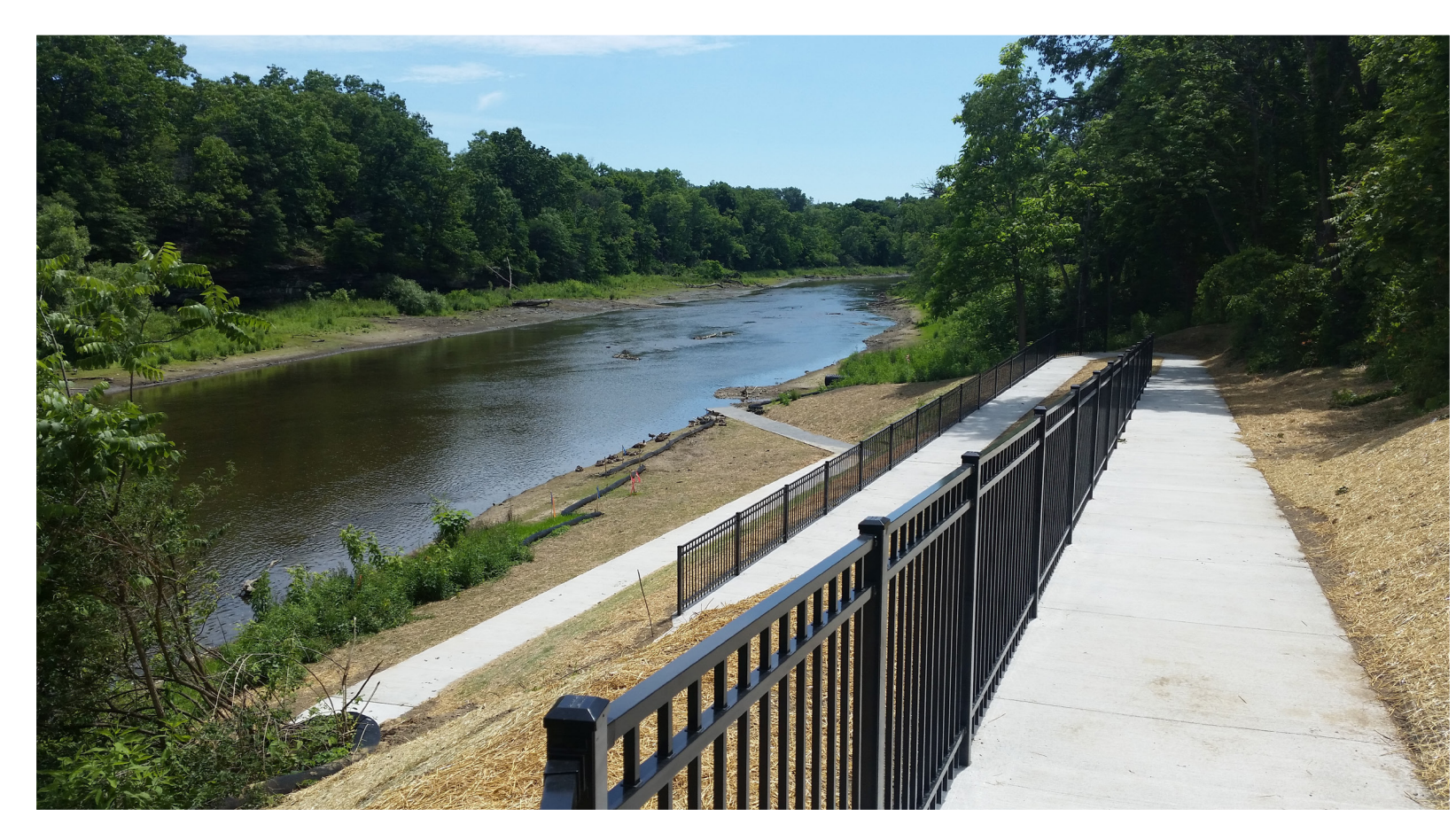
2) River Front Park 2641 Front St, Cuyahoga Falls 0.72 miles to Portage Trail Boat Launch
